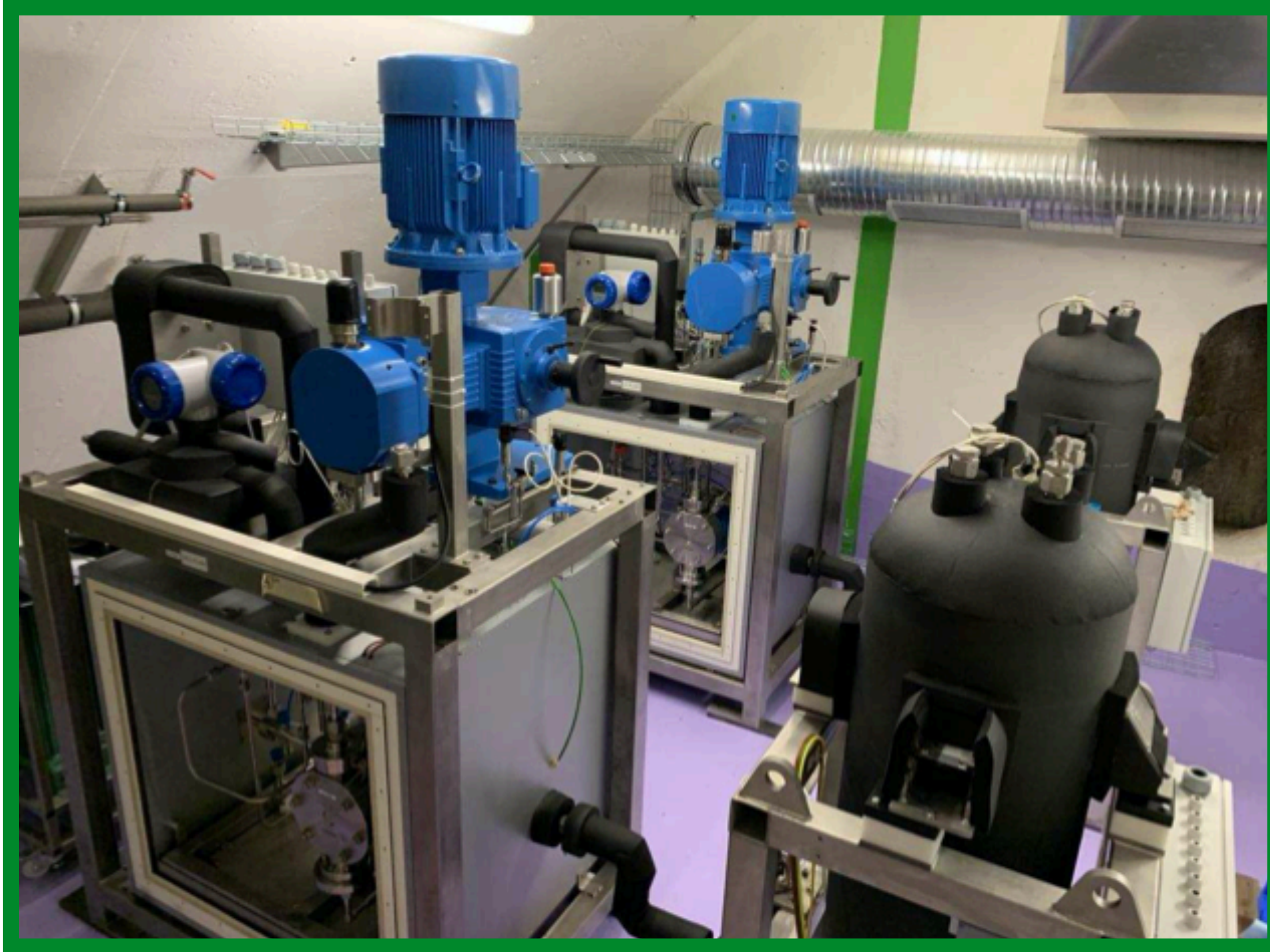
Cooling plant installation
