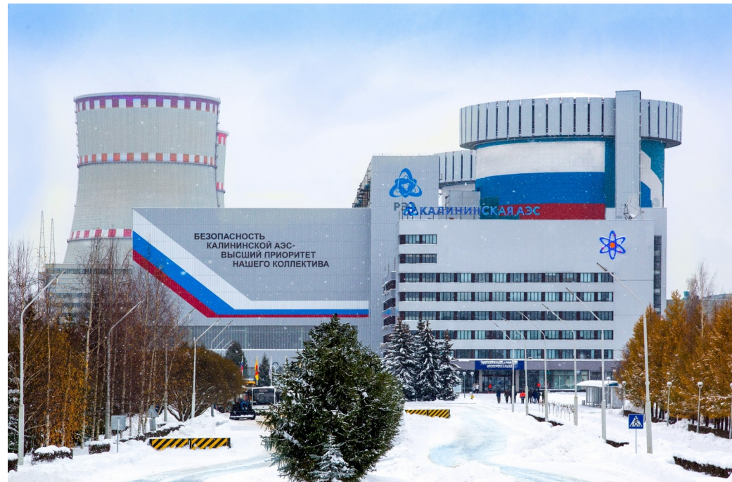
Kalinin Nuclear Power Plant — Udomlya, Tver Region
